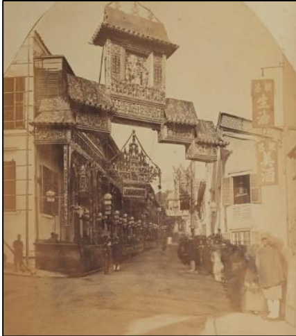
61. THOMSON, John. 'Chinese Street prepared for Illumination', Lyndhurst Terrace, Hong Kong, 1869.
